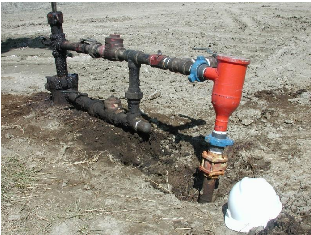
Figure 12. Standard two-inch VF unit installed at well 85-AX-20
