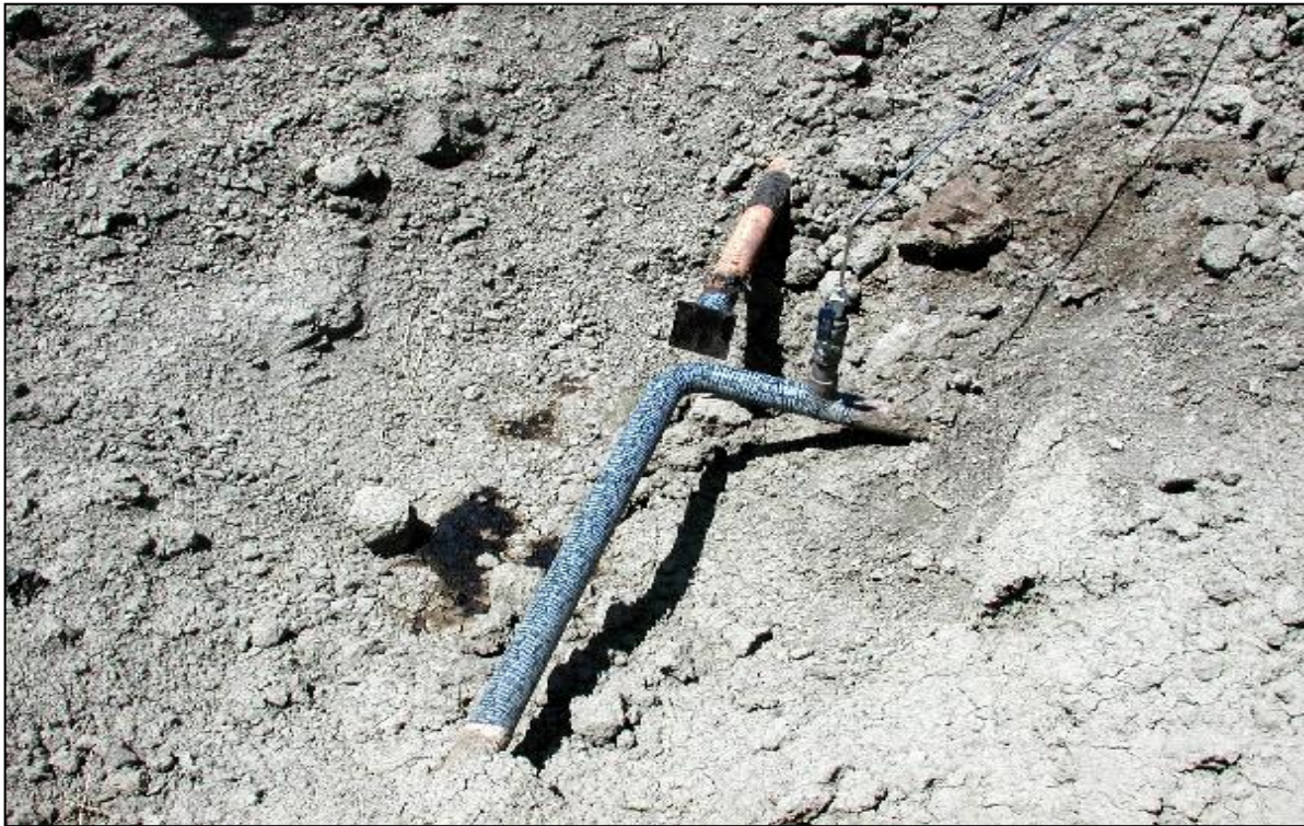
Connection of test manifold to the main Tensleep gathering line, 43-2-TPX-10. Gathering line was dedicated to the Vortex Flow test. Note Barton Pressure Recorder pressure tap.
