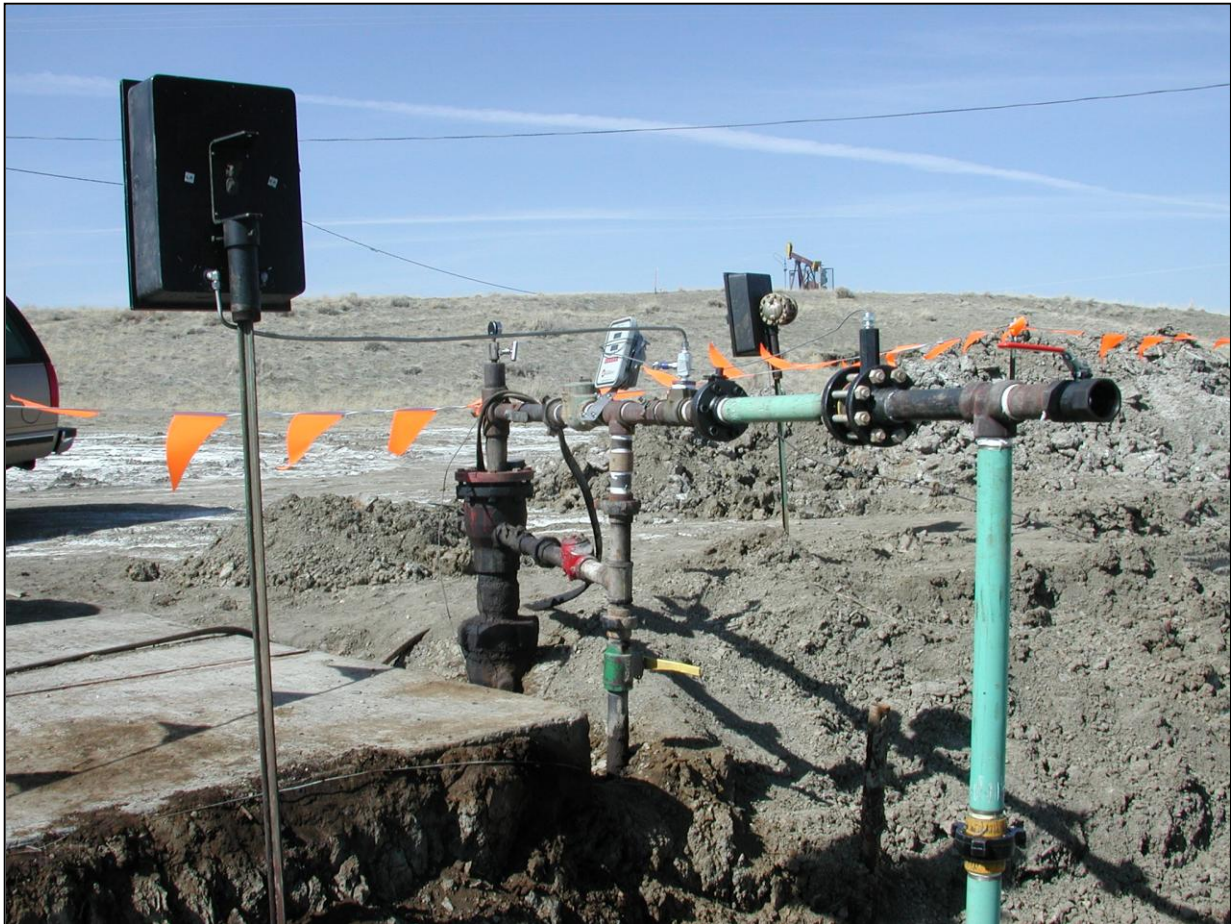
Manifold close-up at 44-1-TPX-10. Black boxes are Barton pressure recorders. Flanged device is the Halliburton flow rate measurement turbine.
