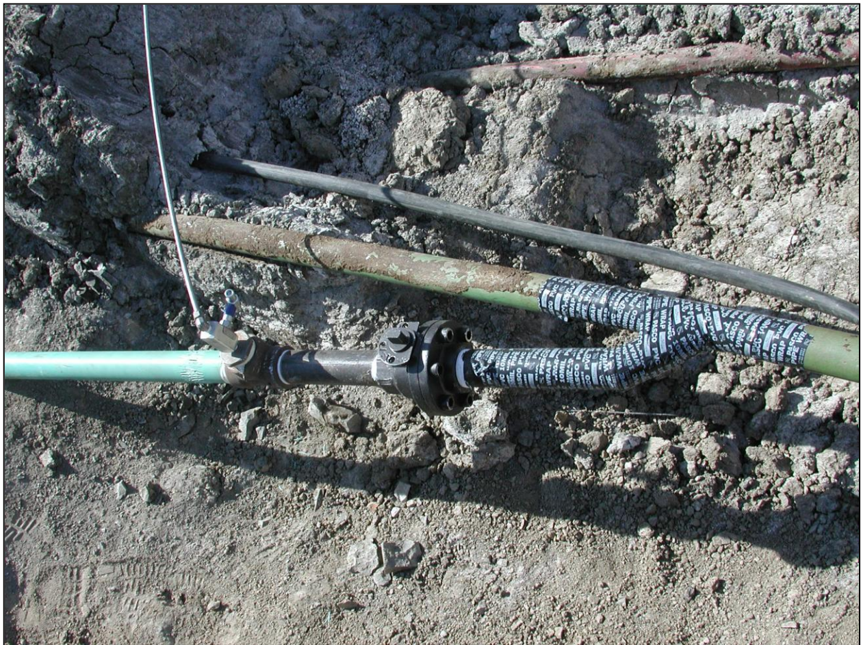
Union of two-inch test manifold with existing production line at well 44-1-TPX-10. Note full bore valve and low side pressure tap for Barton Recorder. Flow is from left to right.
