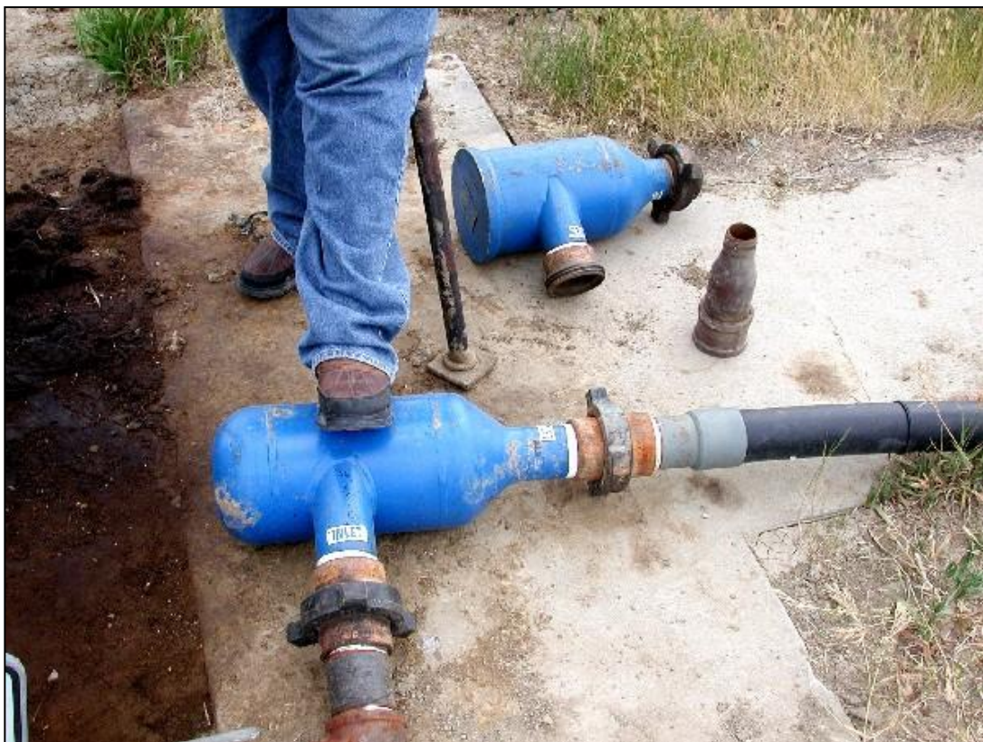
Figure 17. A special domed VF unit installed at 76-MX-3. Standard 90° unit is in the background. The domed unit was designed to meet Canadian specifications.
